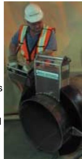
It goes without saying that the operator Demag's both ends of the pipe, before moving onto the next piece. This Demag is performed ahead of welding, by up to 3 or 4 hours. Depending upon the strength of the magnetic field in the middle portion of the pipe, the magnetic field will 'creep' back toward the pipe ends of the pipe, however it can take up to 8 hours for this to occur, so the 3 to 4 hours is a good rule of thumb.
